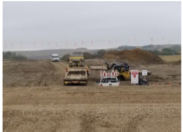
Skidsteer removing matting from flatdeck – SF 34 Sept 11, 2018
