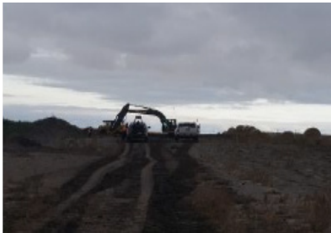
Roach removal and pulling subsoil– SF 47 – Sept 14, 2018
