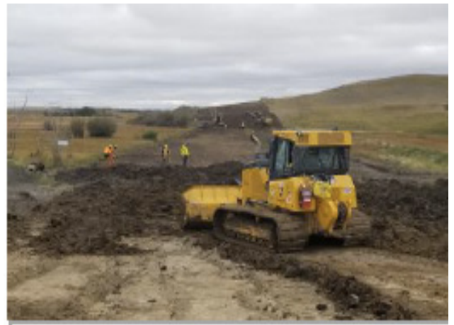
Excavator wetland ramp removal – SF 29 - Sept 14, 2018
