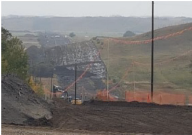
ROW wet and muddy due to rain– SF 29 – Sept 15, 2018
