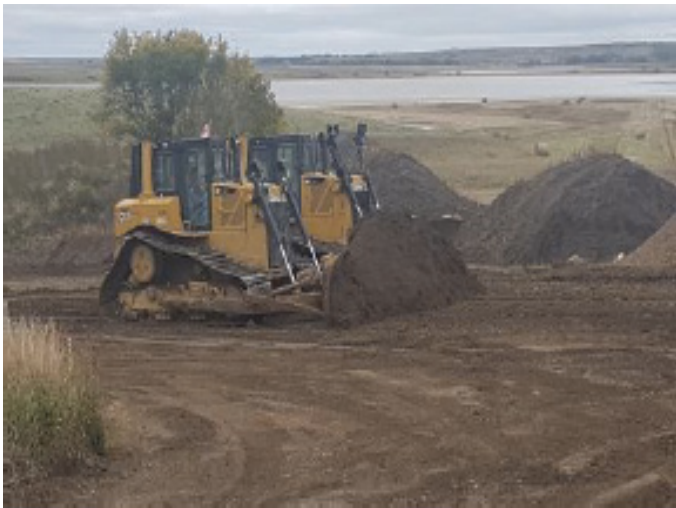
Dozer shaping and contouring subsoil – SF 36 - Sept 13, 2018
