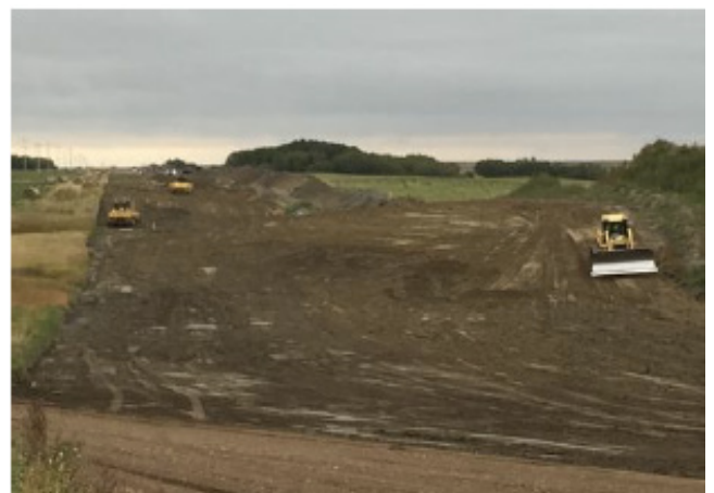
Dozers shaping subsoil – SF 36 –Sept 15, 2018
