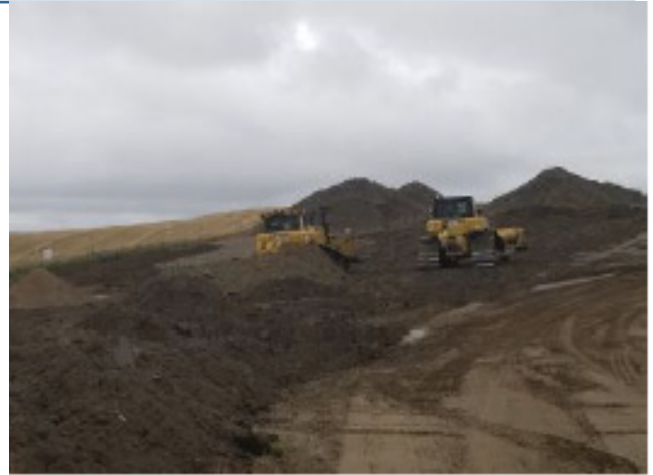
Dozers putting cuts and shaping subsoil – SF 36 – Sept 13, 2018
