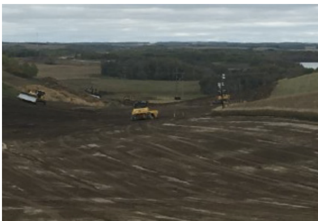
Grader shaping subsoil– SF 35 – Sept 14, 2018
