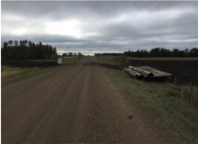
Dirt crew working subsoil on ROW – SF 31 -Sept 10,2018
