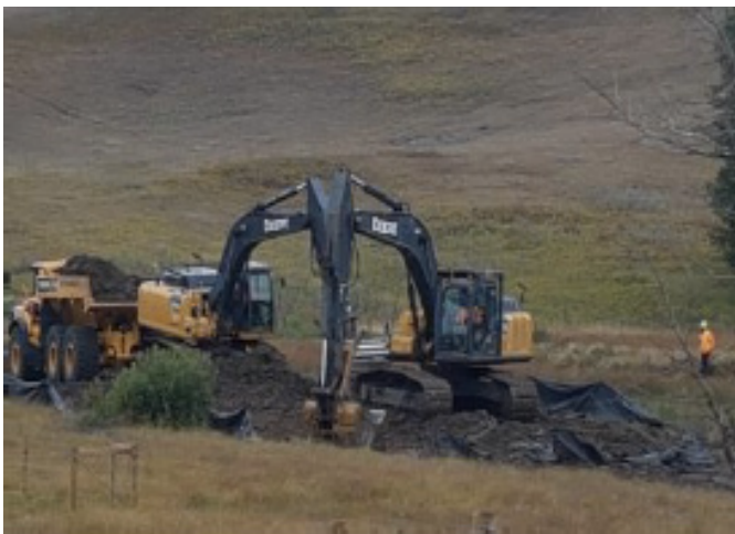
Excavators working on ramp removal – km 41+200 - Sept 12, 2018
