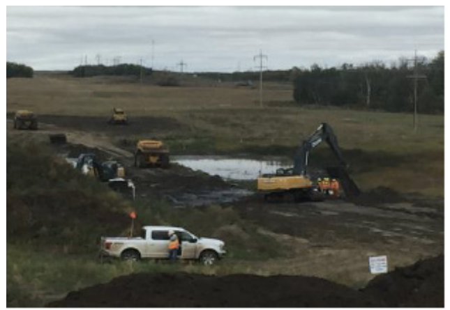
Wetland ramp removal – km 56+600 - Sept 14, 2018
