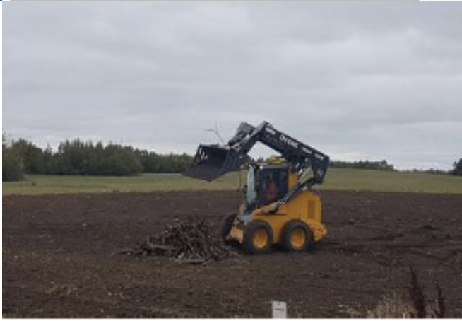
Skidsteer unloading wood debris– km 32+600 – Sept 14, 2018
