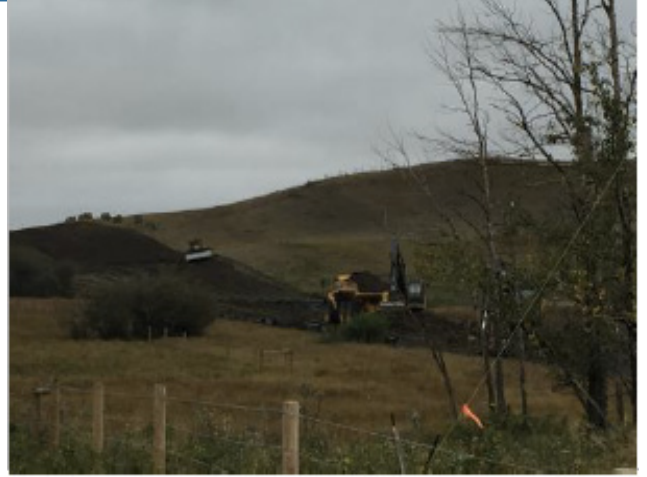
Wetland ramp removal – km 41+200 – Sept 12, 2018
