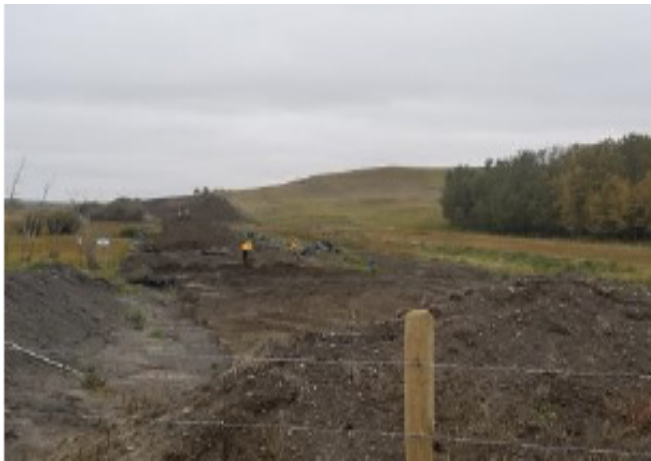
Crews removing geotec from wetland- km 41+200 Sept 11, 2018
