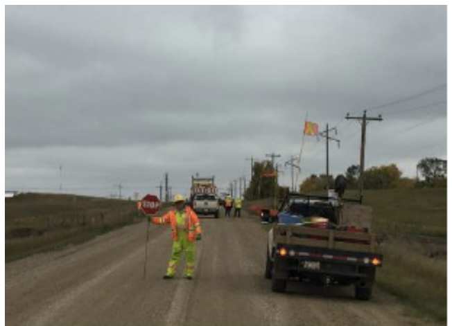
Flagging for traffic control – SF 34&35 – Sept 11, 2018
