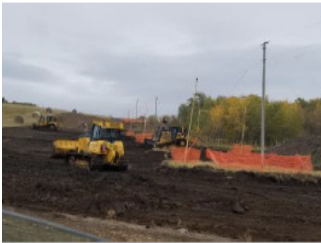
Dozers shaping subsoil and contouring – SF 29 – Sept 15, 2018
