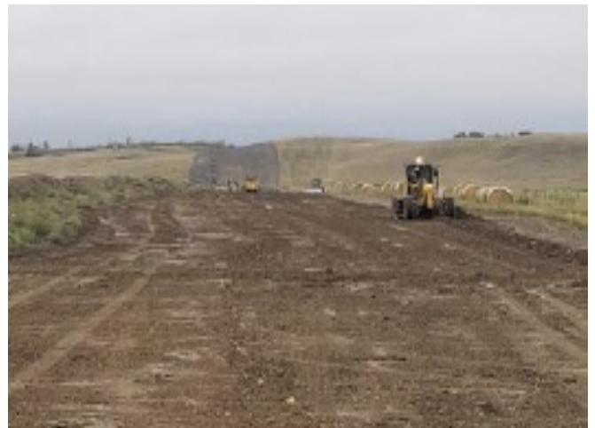
Grader levelling ROW – SF 28 – Sept 15, 2018
