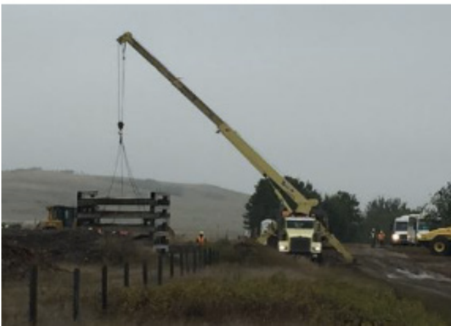
Crane loading bridge brace – km 40+100 – Sept 11, 2018
