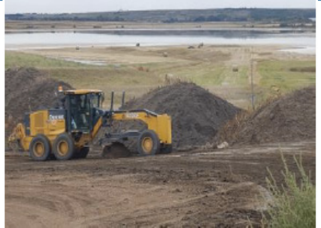
Grader cutting and bulking clay – km 59+000 - Sept 14, 2018
