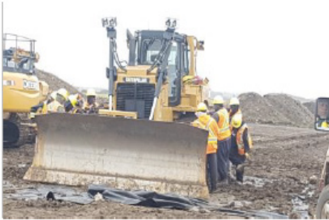
Utility crew rough cleanign dozer - SF 27 - Sept 11, 2018
