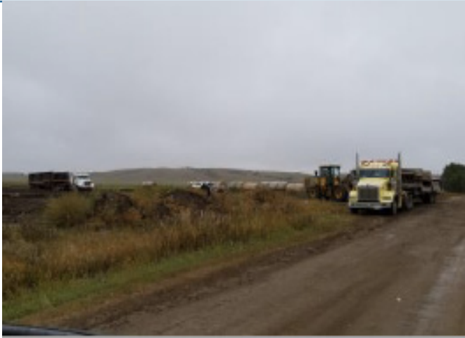
Loading of bridge material – SF 28 - Sept 13, 2018
