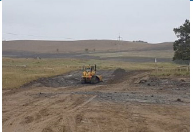
Dozer working on subsoil – SF 36 - Sept 15, 2018
